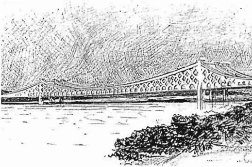
The Puerto Rico Bridge, prestressed concrete shell design, 500 meter span, by Center for Environmental Structure and T. Y. Lin International, 1995
