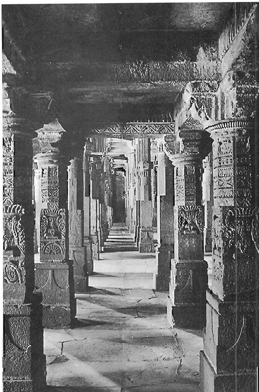
Ahmedabad. Ahmad Shah's mosque, interior. 1414
