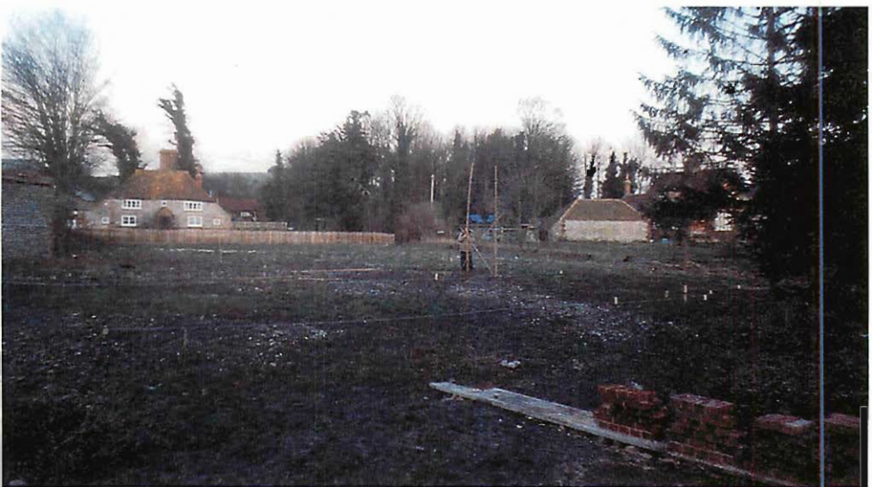
The site, two flint cottages, and, on the right, my earliest mockups of brick and flint where I first tried to find combinations of material that felt right on that land
